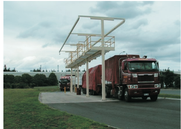
A truck tarping station enables a driver to use fall prevention equipment
