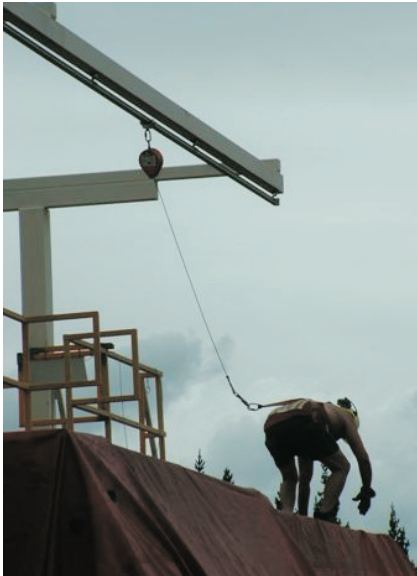
Tarping structures on sites with harnesses including emergency response
